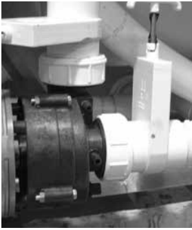
Slice Valve and Pump Union
