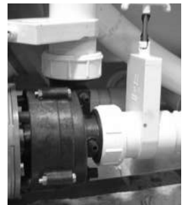
Slice Valve and Pump Union
