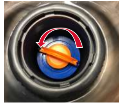
Turn Filters Counter-clockwise to Remove
