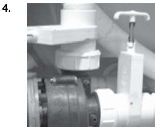
Slice Valve and Pump Union
