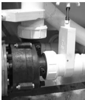
Slice Valve and Pump Union
