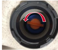
Turn Filters Counter-clockwise to Remove
