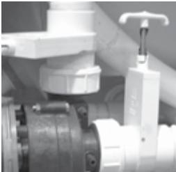
Slice Valve and Pump Union
