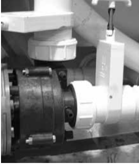
Slice Valve and Pump Union
