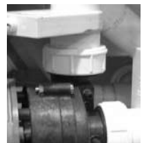
Slice Valve and Pump Union
