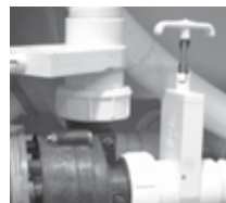
Slice Valve and Pump Union
