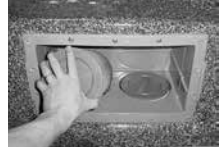
Turn Filter Counter-clockwise to Remove
