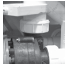
Slice Valve and Pump Union
