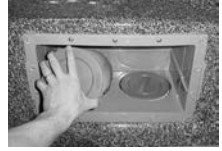
Turn Filter Counter-clockwise to Remove
