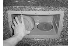
Turn Filter Counter-clockwise to Remove
