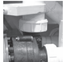
Slice Valve and Pump Union
