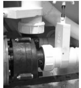
Slice Valve and Pump Union
