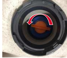
Turn Filters Counter-clockwise to Remove
