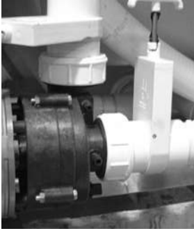
Slice Valve and Pump Union
