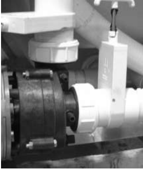
Slice Valve and Pump Union
