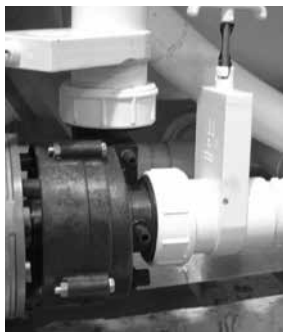
Slice Valve and Pump Union
