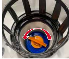
Turn Filters Counter-clockwise to Remove
