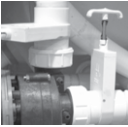
Slice Valve and Pump Union
