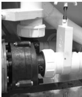
Slice Valve and Pump Union
