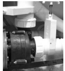
Slice Valve and Pump Union
