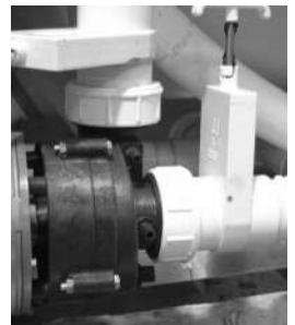
Slice Valve and Pump Union
