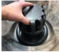
Pull Up to Remove Floater Assembly
