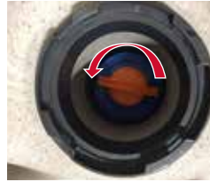
Turn Filters Counter-clockwise to Remove
